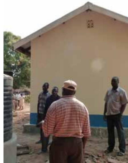
The village residents also participate in the construction work.
